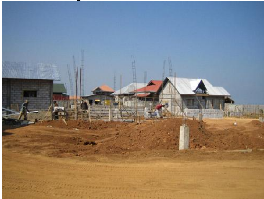
Figure 3.23: Construction of Houses by skilled labor in Brgy. Sto. Domingo
