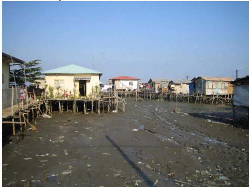
Figure 3.25: Some make-shift houses along the coast in Brgy. Capunitan
