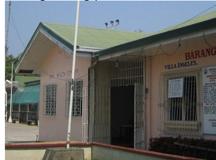
Figure 3.14: Barangay Health Center incorporated in the Villa Angeles Barangay Hall
